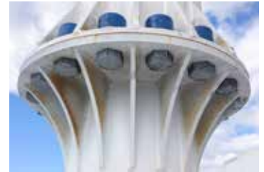
Nord-Lock has taken on a crucial role with the SeaTwirl prototypes, delivering both washers and Superbolts.
